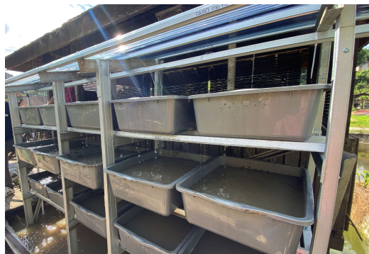
Figure 7. Practical Stage: Water Flow Installation
