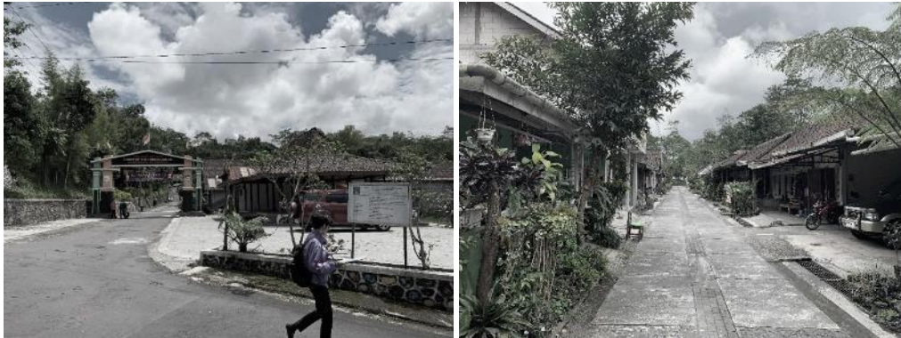
Figure 3. The housing conditions and infrastructure of Karang Kendal.
