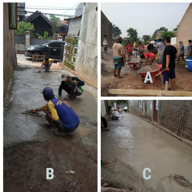
Figure 7. The process of implementing road concrete (A) the process of making concrete with a manual concrete mixer, (B) the process of leveling the concrete mix, (C) the condition of the concrete after it has been leveled.
