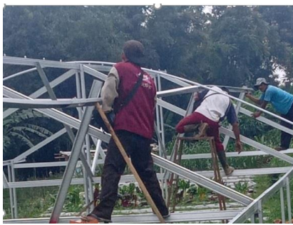
Figure 16. Mentoring on green house construction
